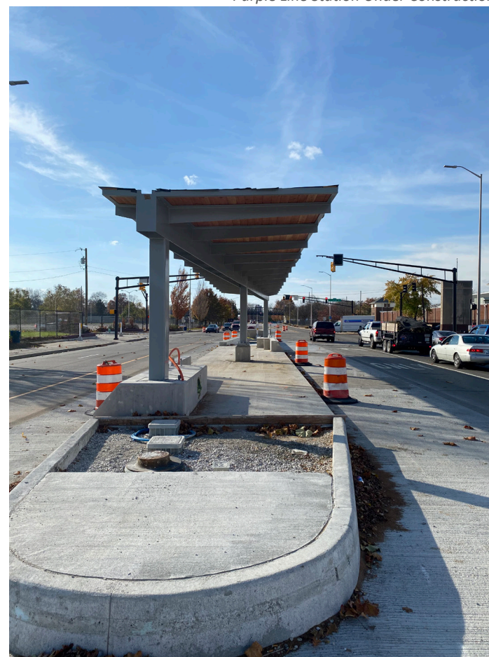
Purple Line Station Under Construction
